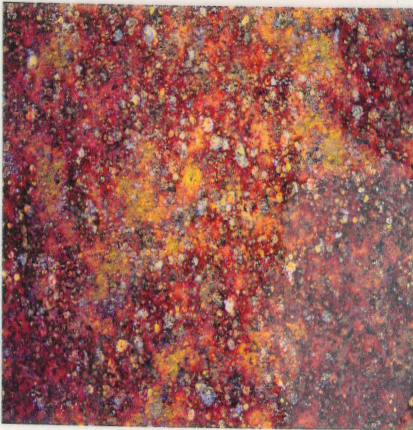
Before Surface Preparation.
