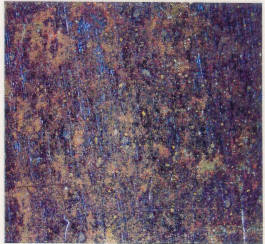
After Surface Preparation.
